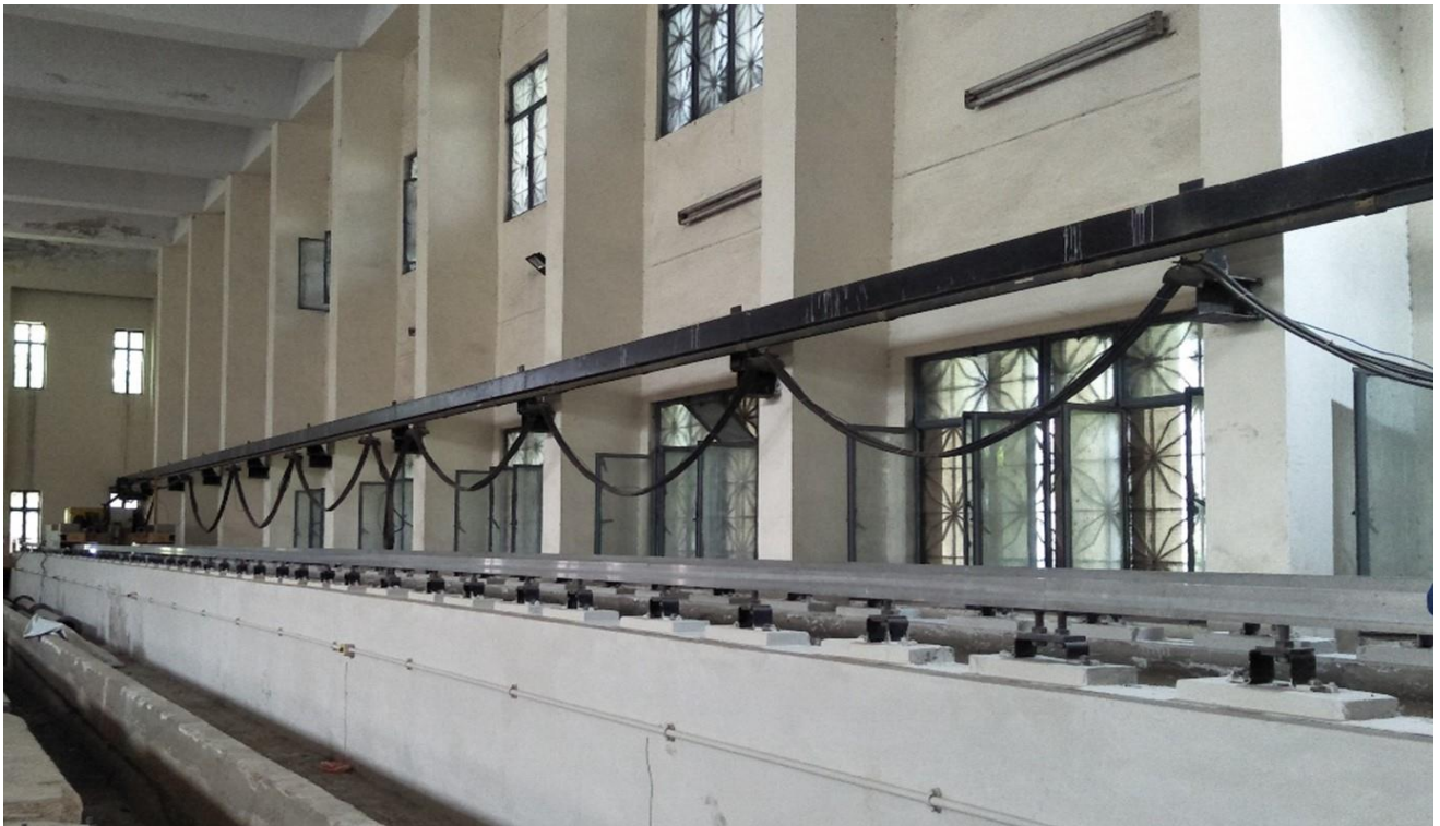
Figure 1: Channel and rail track of trolley
